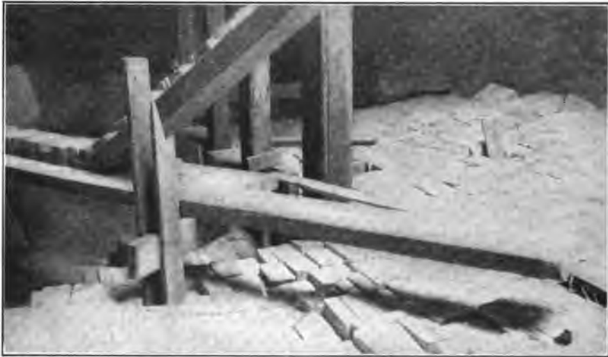
FIG. 150.—Hold of schooner shown in Fig. 149; note bottom of chute and method of stowing the brick. The breakage on this shipment was practically nil.
